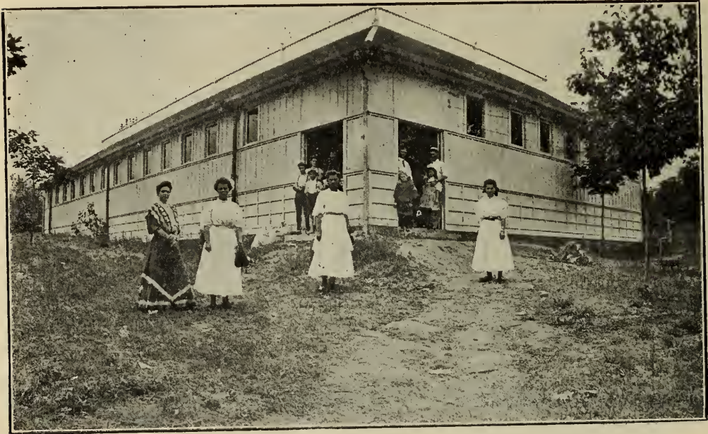
BATH HOUSE AND SWIMMING POOL.
