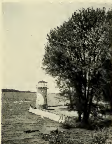
The Lake Wall and Chautauqua Lighthouse Erected 1940
